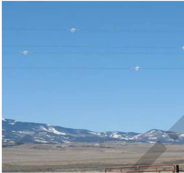
Plate 1: Electricity line marked with swan flight diverters
